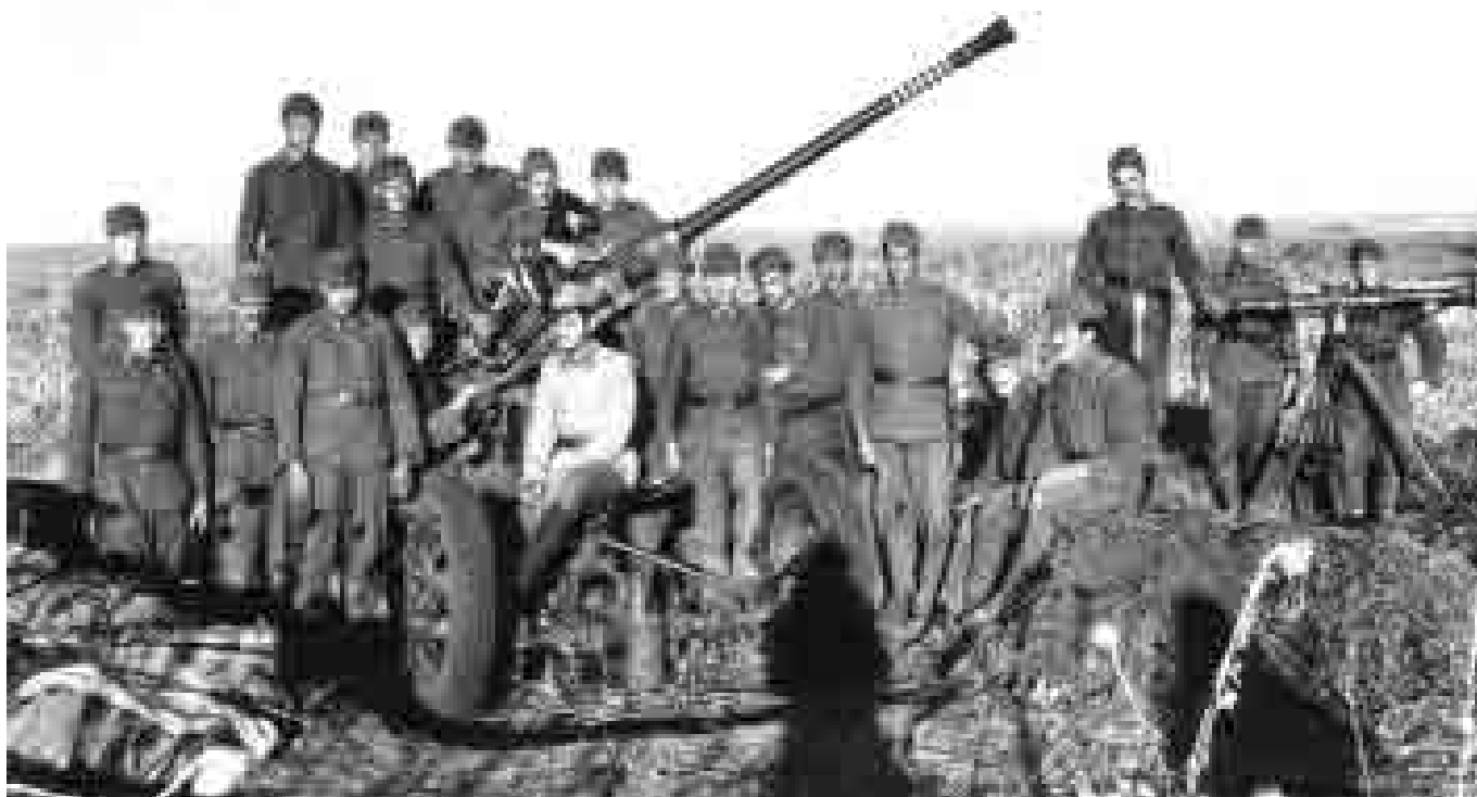
Powerful armament of Hungarian AA defense. Swedish 40mm caliber Bofors. VVKJ Blenheim crews from 8.BP remembered those by their powerful performance ( Csaba Besce coll )
